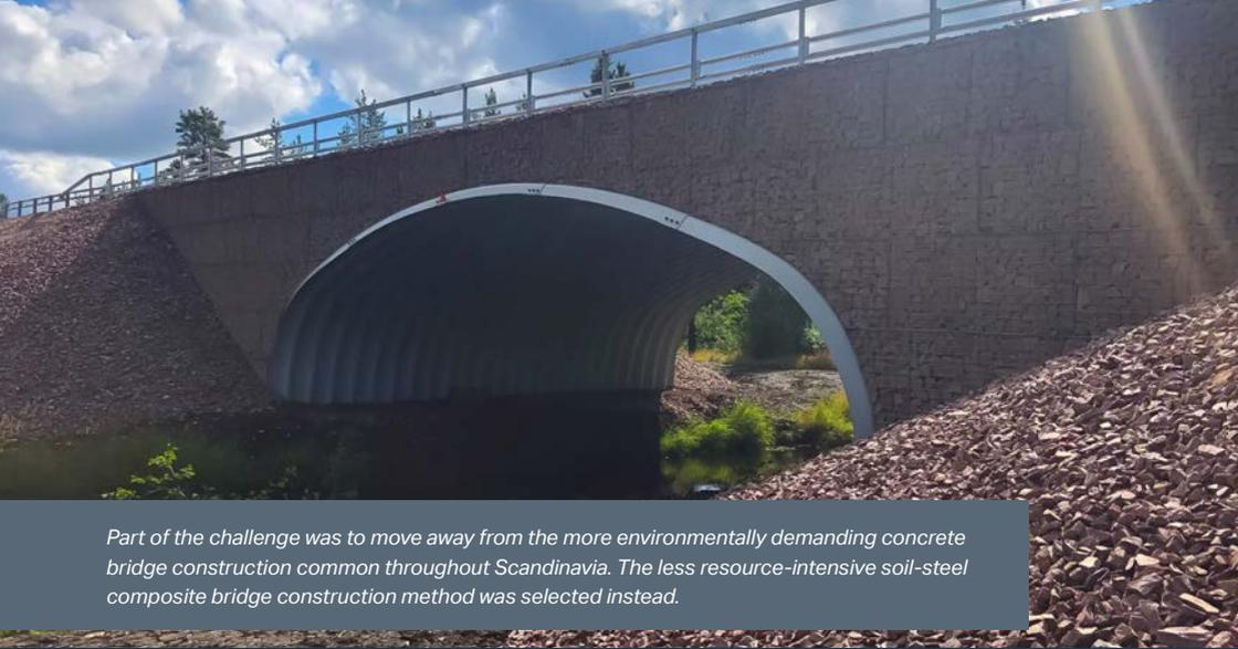
*Part of the challenge was to move away from the more environmentally demanding concrete bridge construction common throughout Scandinavia. The less resource-intensive soil-steel composite bridge construction method was selected instead.*
