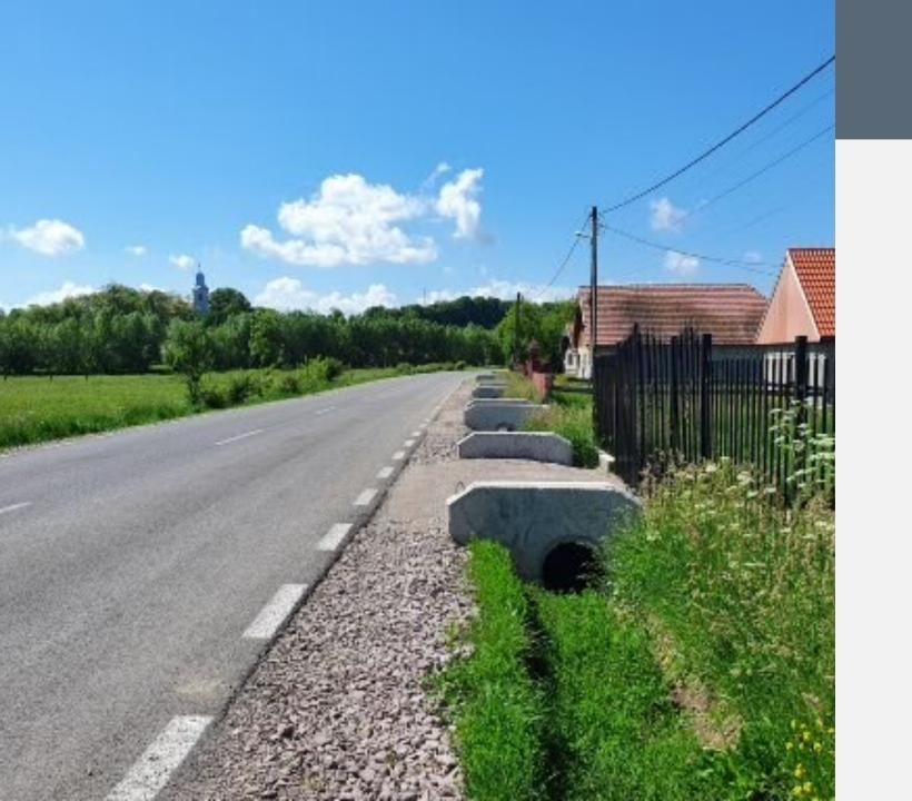
Culverts for access to properties provided with prefabricated reinforced concrete headwalls.
