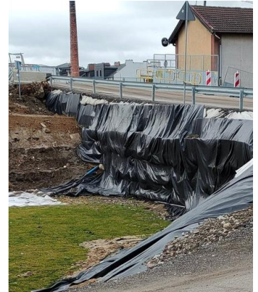
Figure 8. Bypass temporary construction - facing.
