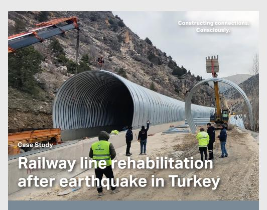
ViaCon Türkiye worked on post-earthquake renovation of steel corrugated culverts, bridges and tunnels on 4 railway lines.
