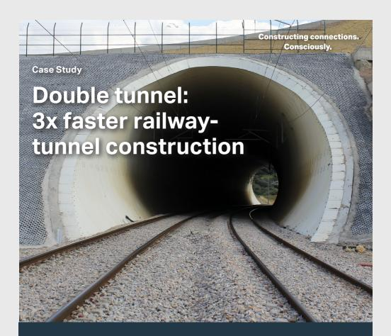
ViaCon corrugated steel solution cuts down construction time on a second tunnel in Algeria. Corrugated steel solutions add flexibility to tunnel construction projects when time is of the essence.
