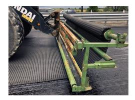
The result: a stronger pavement structure with significantly reduced risk of reflective cracking. Thanks to the geogrid's ease of handling and seamless integration into asphalt paving workflows, installation was completed efficiently and with minimal disruption.
