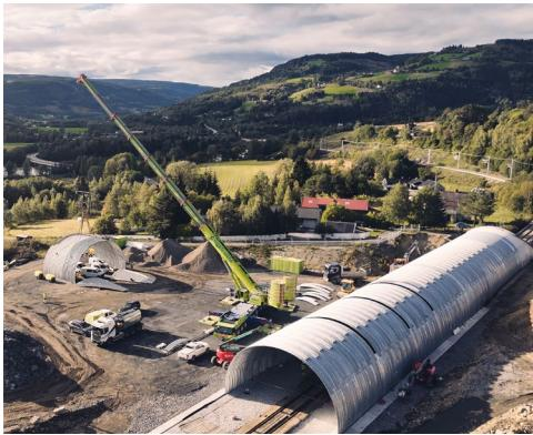
and placement of the soil–steel sections within a single 72-hour train stoppage window. Crane operations were planned with Nordic Cranes and backfilling was executed by AF Anlegg with subcontractor Løype Anleggsdrift AS, ensuring continuous progress throughout the possession.
